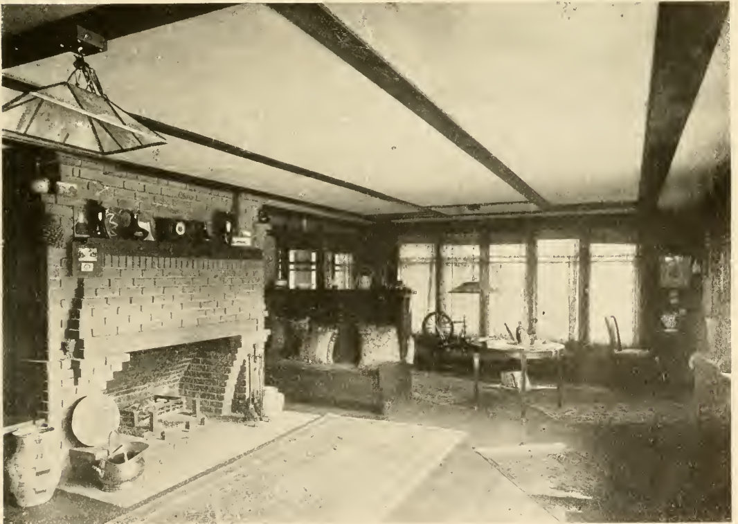
A Charming Craftsman Interior Showing Clinker Brick Fireplace with Lintel of Fireproof Wood
